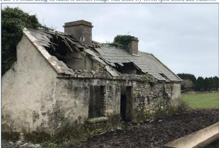
Plate 4-6 North facing elevation of derelict cottage with partially collapsed roof.
