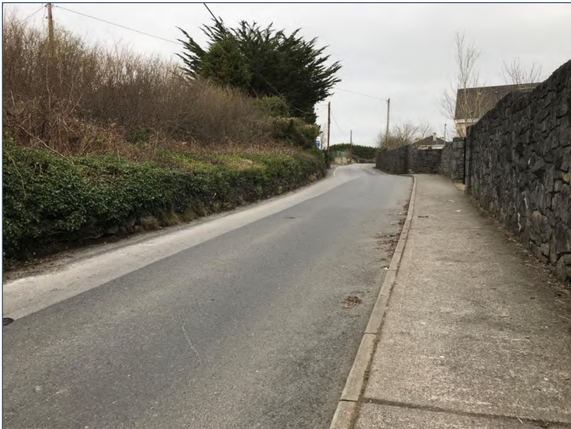
Plate 5-6 The site boundary extends to include the local road to the south classified as Buildings and Artificial Surfaces (BL3).
