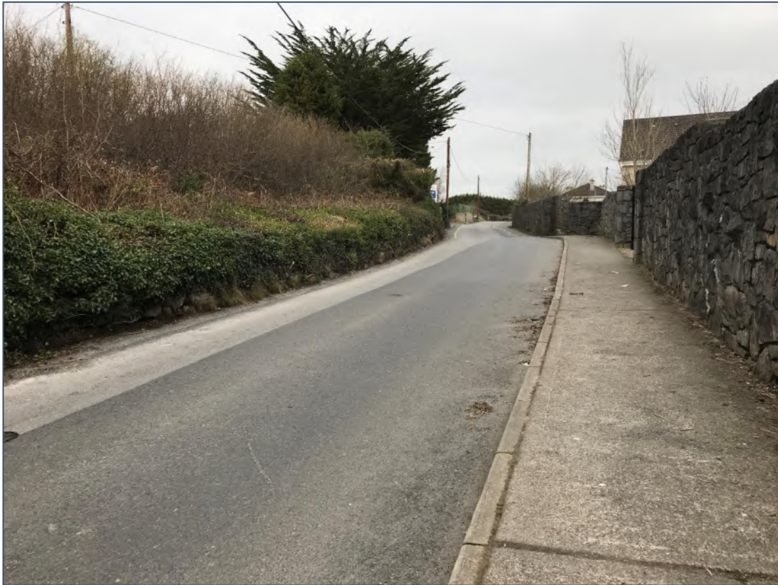
Plate 2-6 The site boundary extends to include the local road to the south classified as Buildings and Artificial Surfaces (BL3).
