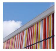
Coloured Fibre Cement cladding
