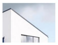
Flat roof with sloping parapet
